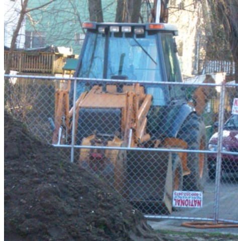
Site work at Watertown Community Housing’s 1060 Belmont Street project
