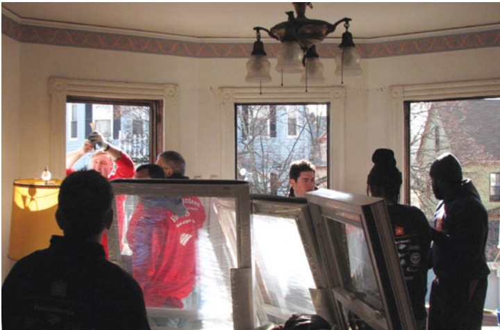
Nuestra CDC Partners with YouthBuild Boston to provide weatherization assistance and training through the Partnership for Greening Blue Hill Avenue.
