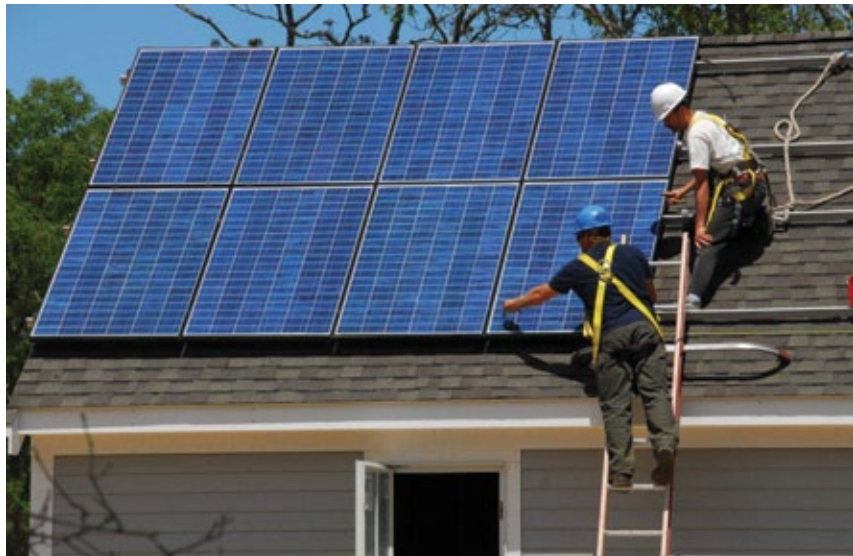
Solar panels, like these installed recently on a CDP housing development, will conserve energy and create revenue in the Real Return Initiative.
