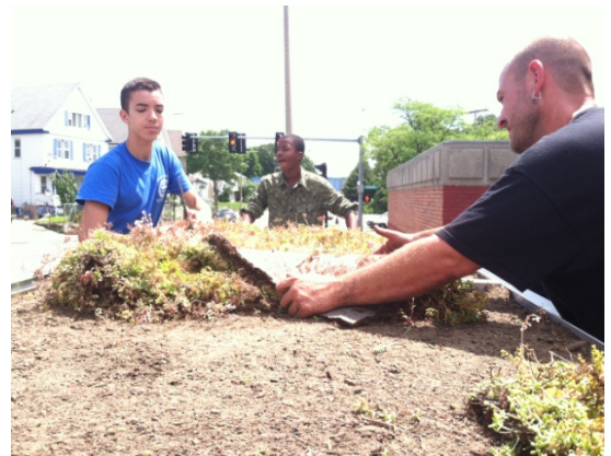
Installation of green roof on Talbot Avenue in Dorchester.
