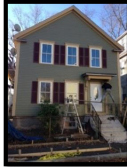
43 Pleasant Facade Restoration
